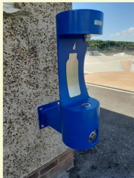
Photo above - the popular water bottle refill station at The Salts.
