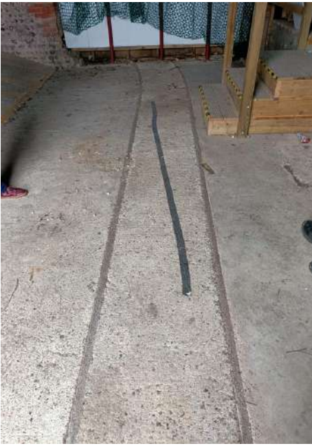
Narrow gauge railway track
