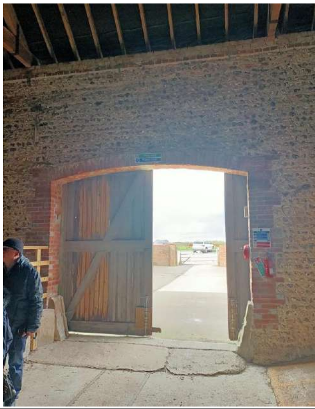
Main Barn looking to courtyard
