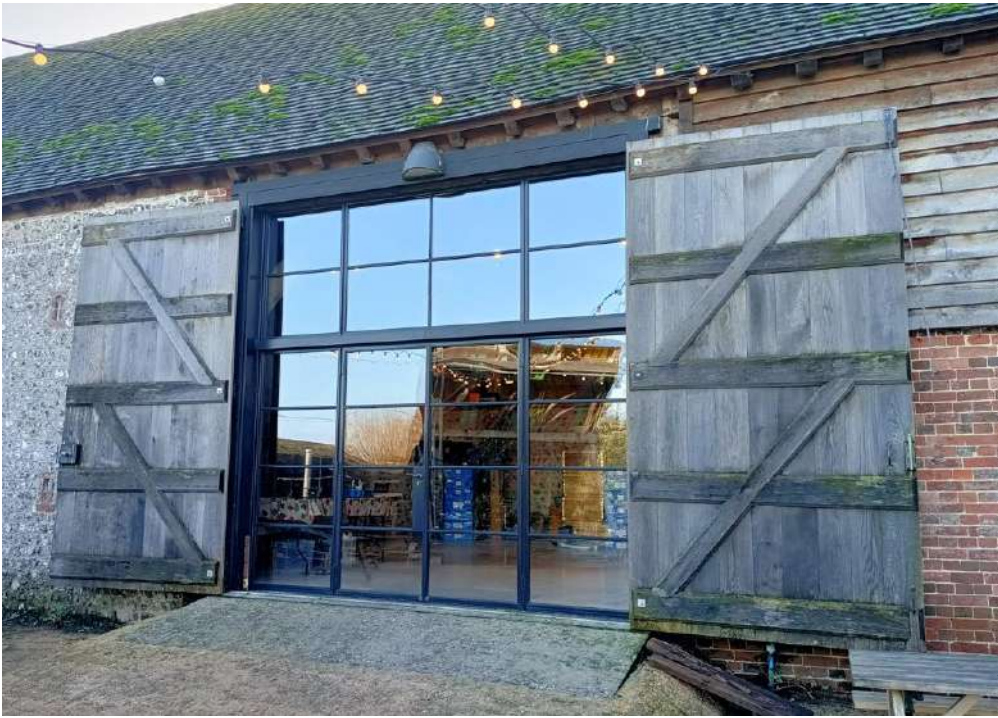
Main barn entrance
