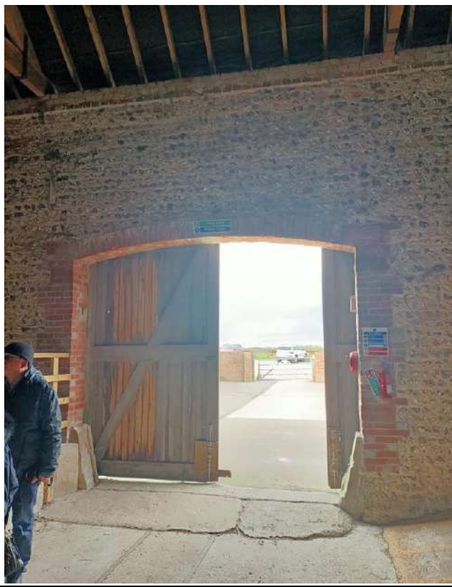
Main Barn looking to courtyard
