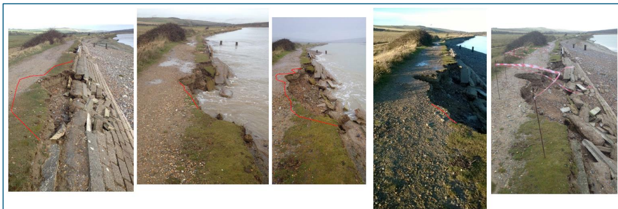
Figure 3.2. Erosion of the southern end of the east embankment between March 2016 and November 2016. The red line represents the approximate position of the erosive scarp in the succeeding photograph. Photographs courtesy of Uwe Dornbusch
