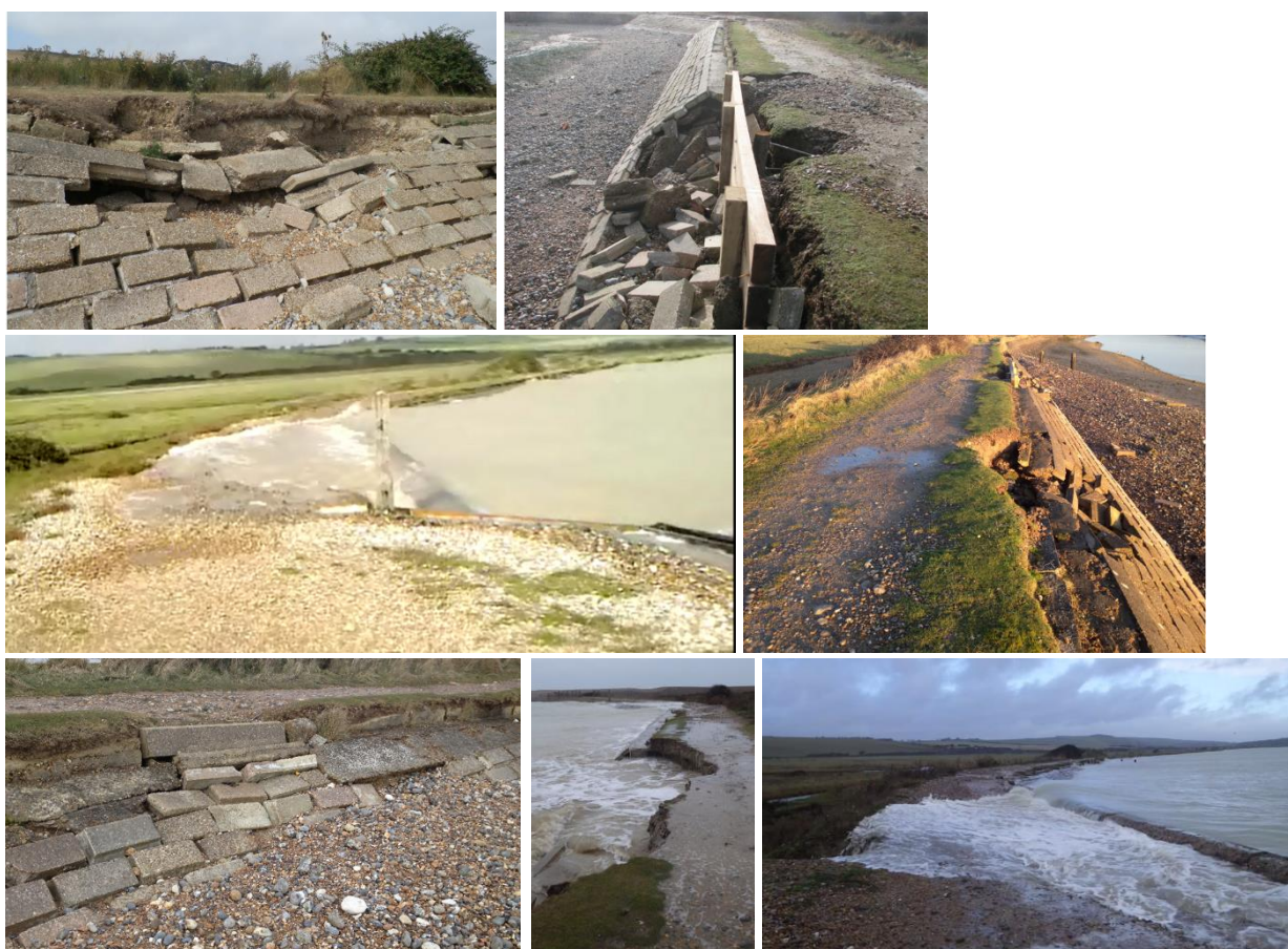
Figure 3.1. Photographs of damage, repair and overtopping along the southern end of the east embankment between 2013 and 2016. Damage 18 th August 2013 (top left), Repair 5 th February 2014 (top right), Overtopping 9 th October 2014 (centre left), Damage 13 th January 2016 (centre right), Repair 28 th March 2016 (bottom left), Damage 17 th November 2016 (bottom centre), Overtopping 17 th November 2016 (bottom right). Photographs courtesy of Uwe Dornbusch
