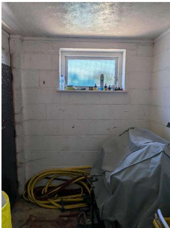
Toilet block interior
