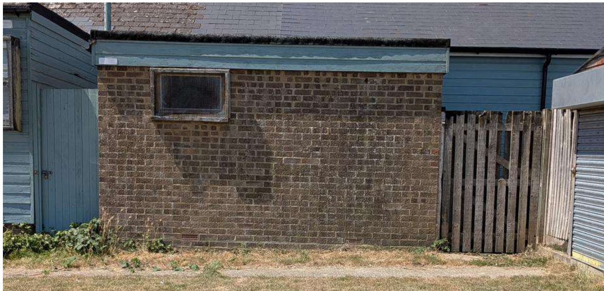
Toilet Block Exterior
