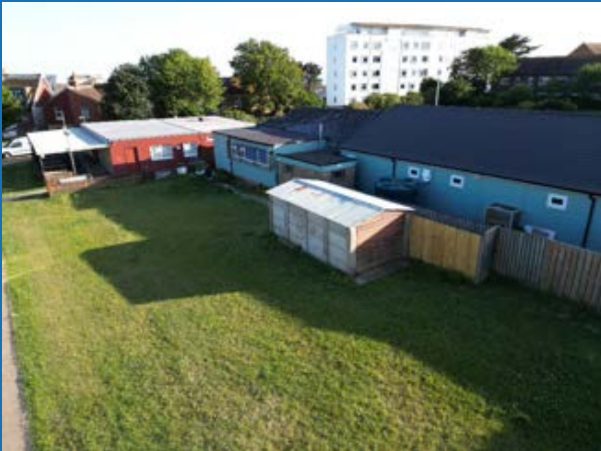
STFC Clubhouse/Pergola + Garage
